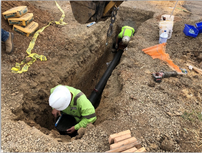
Crews at Yosemite & G St performing a hot tap to install a new fire hydrant
