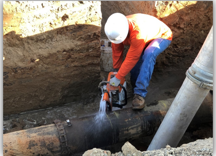
Tee Installation for Sage Creek Subdivision
